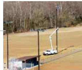
Poles above 40' Mounting Height are supplied in two sections, to be joined on site as shown.
