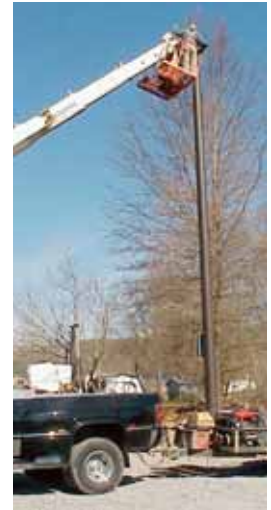
Poles above 40' Mounting Height are supplied in two sections, to be joined on site as shown.
